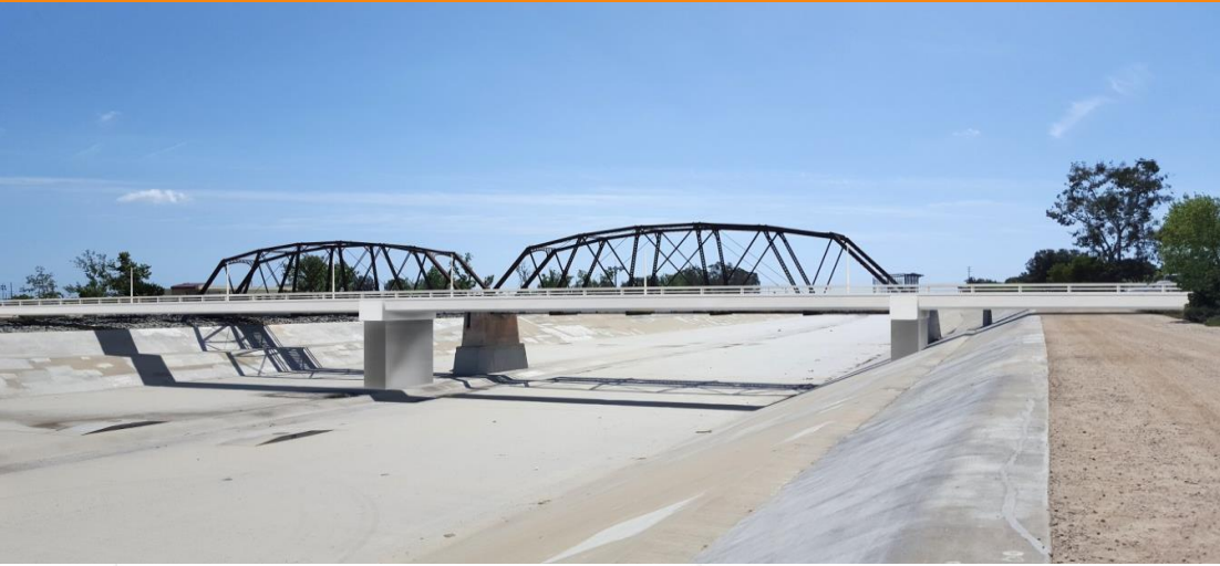
New Trail Undercrossing
